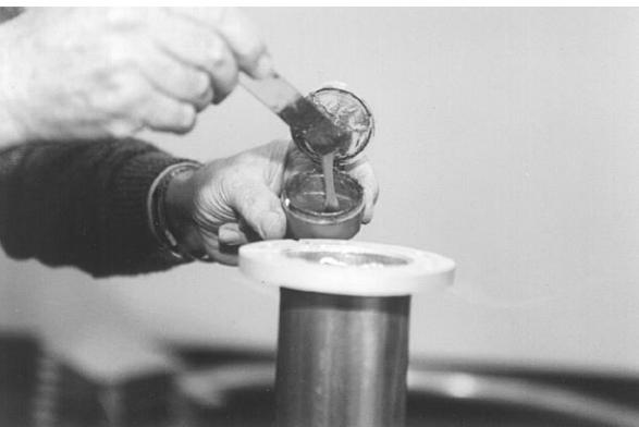
Spread the provided anti-oxidant paste on the flange.
