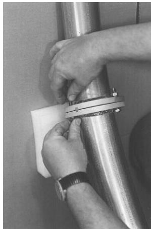
After spreading the anti-oxide paste in the grooved flanges, unite the flanges and install the bolts and nuts.
